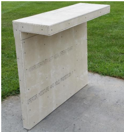
Split Bar Counter With Cement Board
