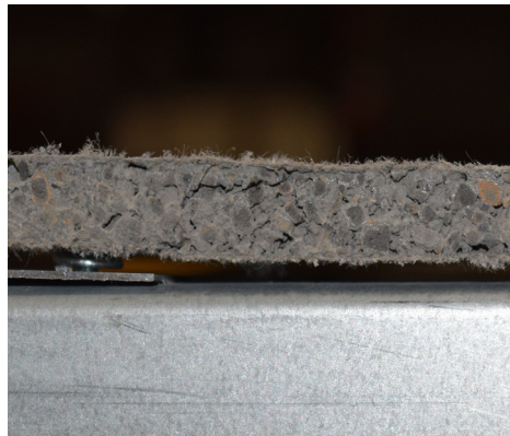
Their panels with cement board attached to frames assembled with screws creating a gap.
