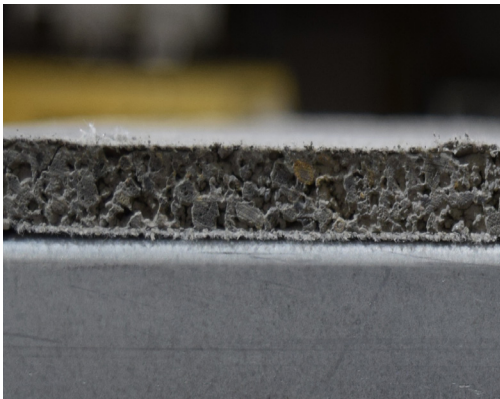
Rapid Panels™ with cement board attached to fully welded frame. Cement board sits flat.
